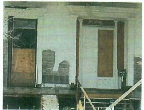
Beauvoir (April 2006), detail of front door and windows.
