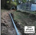
Work has been going on to finalize the installation of the new sewer plant. Recently new effluent lines have been dug in, tanks & air lines inspected, etc and plans are in place to put the new unit online, October 15th, 2022.
