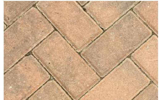
Actual Lowcountry Paver driveway after 10 years!
