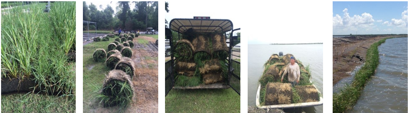
Photos 4-8 Pre-vegetated Matrix Strips Planted, Rolled, Loaded, Delivered, Installed
