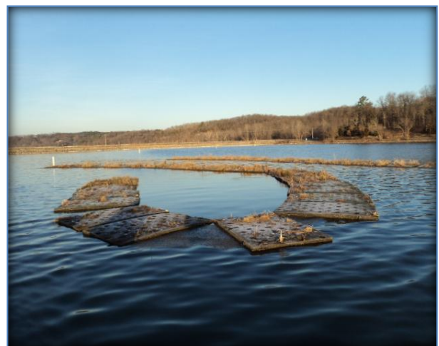
Figure 21 Loose sections of floating islands January 19, 2012.
