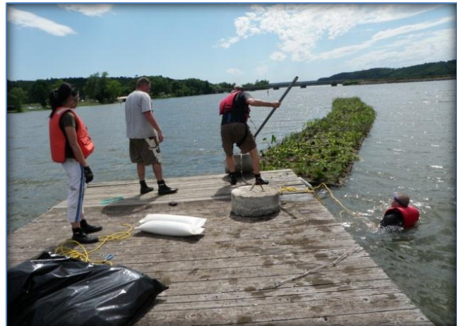
Figure 2 Anchoring the first 100' chain.
