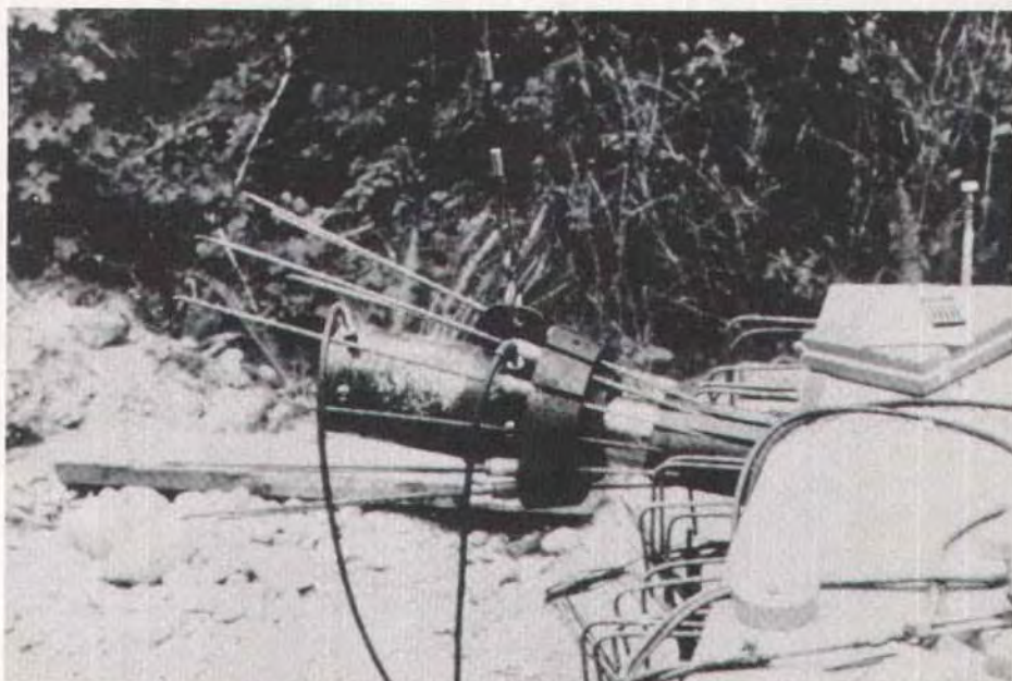
Fig. 16. Jacking was performed on one end of each girder individually.
