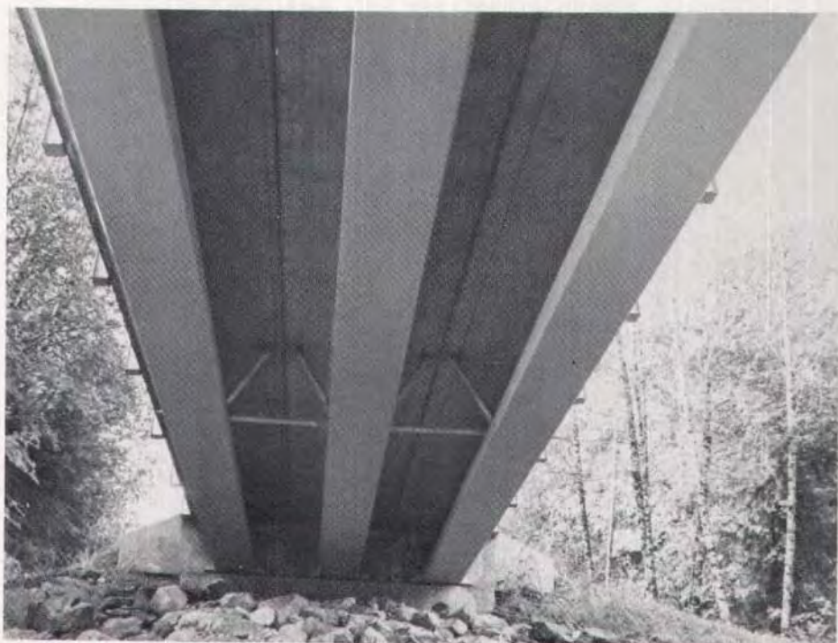
Fig. 19. Galvanized steel pipe diaphragms were used at maximum positive moment locations.
