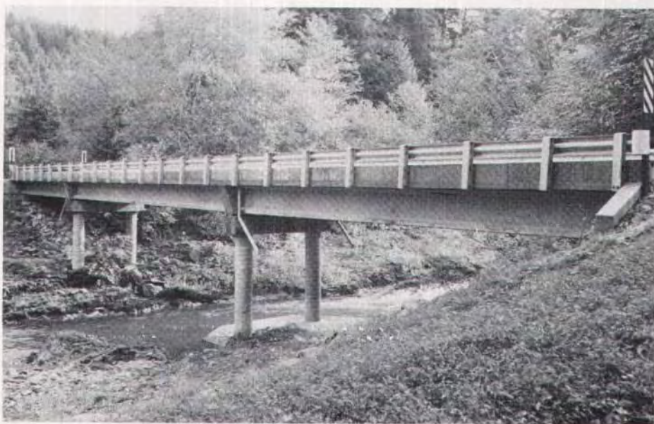
Fig. 20. Tapering the ends of the raised cross beams and providing sloped stiffeners at the top of the guardrail posts do their part in enhancing the aesthetics of the bridge.
