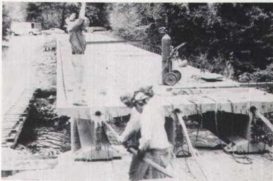
Fig. 15. The center span of the old timber bridge was used as a temporary construction bridge. The high termination anchorage of the post-tensioning is shown. Duwayne Hankins, project engineer from Concrete Technology, directs the post-tensioning operation.
