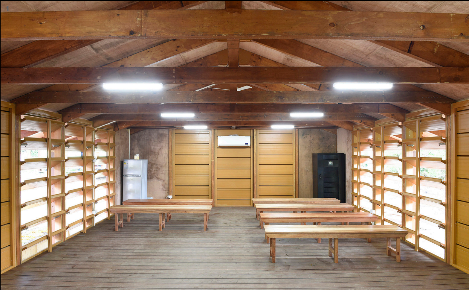
1. Classroom, Tanna Island VU One of 14 Nakamal (multi-purpose community) flat pack buildings delivered to 12 remote villages. 2. Classroom, Tanna Island VU Large overhangs & full height shutters control privacy, permit ventilation even in hot humid rainy conditions. 3. Research Masters: Pilot Project, Gracemere AU Ken's research into the applied use of laminated timber in commercial construction was a leader in Australia. High level louvres permit natural ventilation when the building is not in use. Images include experience gained under engagement with former practices.
