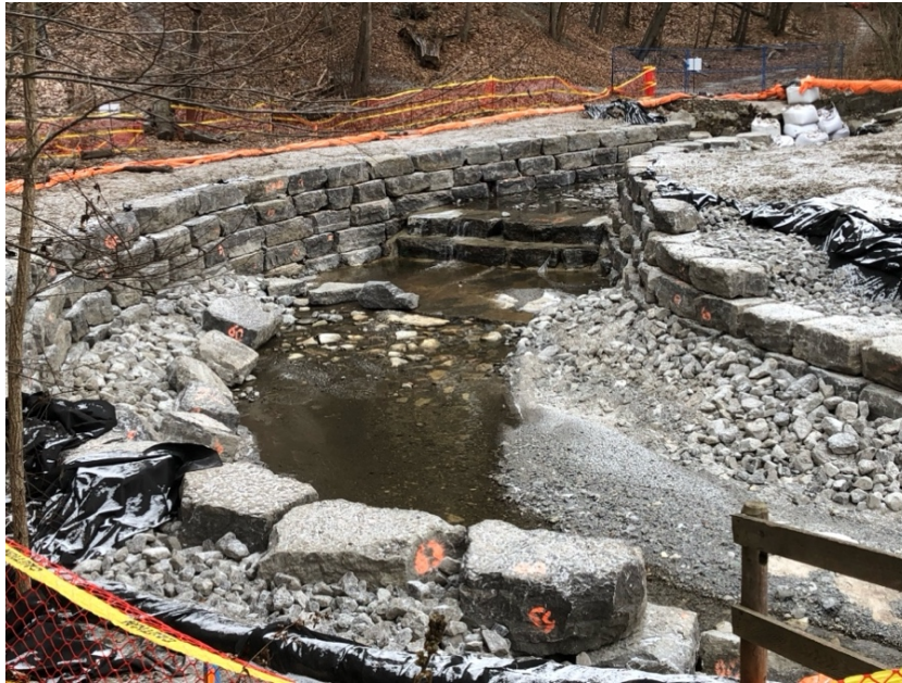
Current TRCA design example (project below Summerhill). Note the substantial widening of the stream, the energy-reducing waterfall, and protected armour-stone (granite block) walls. All necessary to withstand 21 st century storms.
