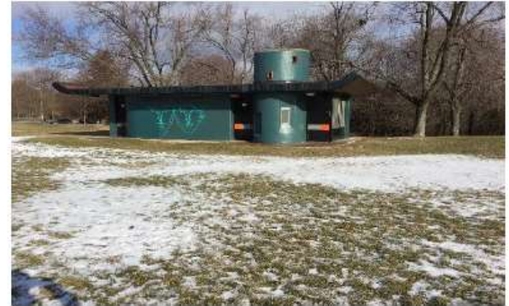
New public washroom
