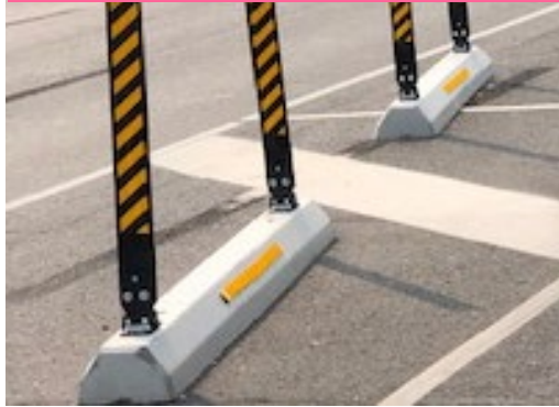
2m between curbs + posts & reflective strips
