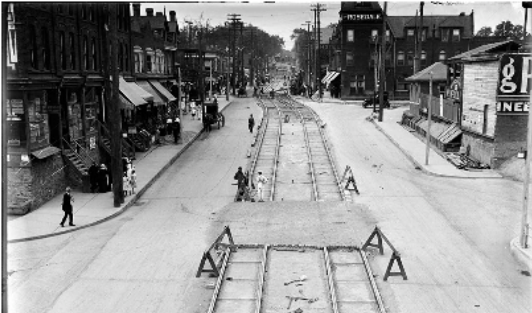
1916 laying new track looking North from Birch Ave Note Rosedale Hotel
