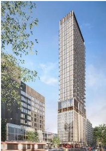
1 St. Clair Avenue West
