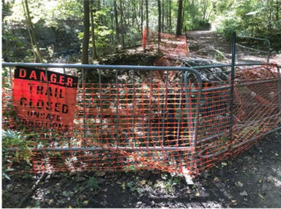
Stream bank erosion
