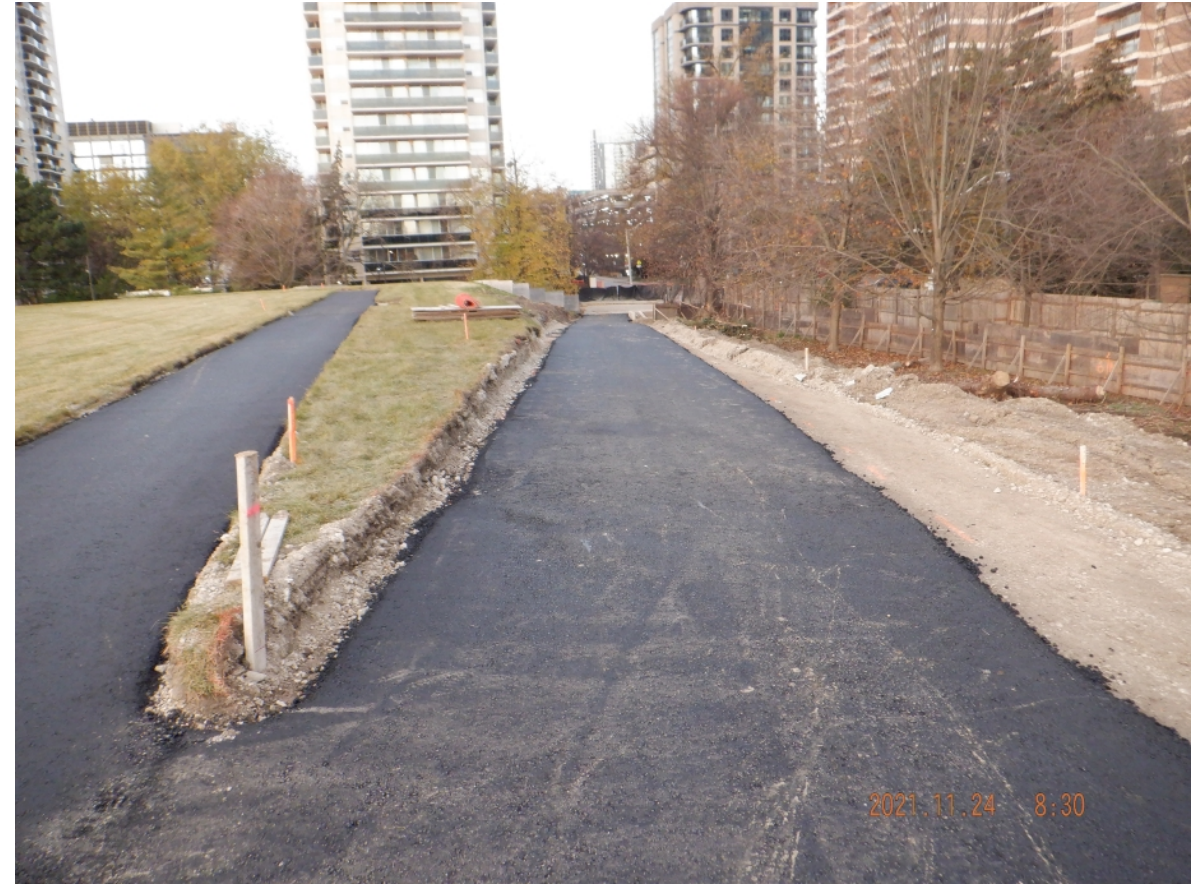
Ramp from Rosehill entrance node to Upper Pathway (View looking west)
