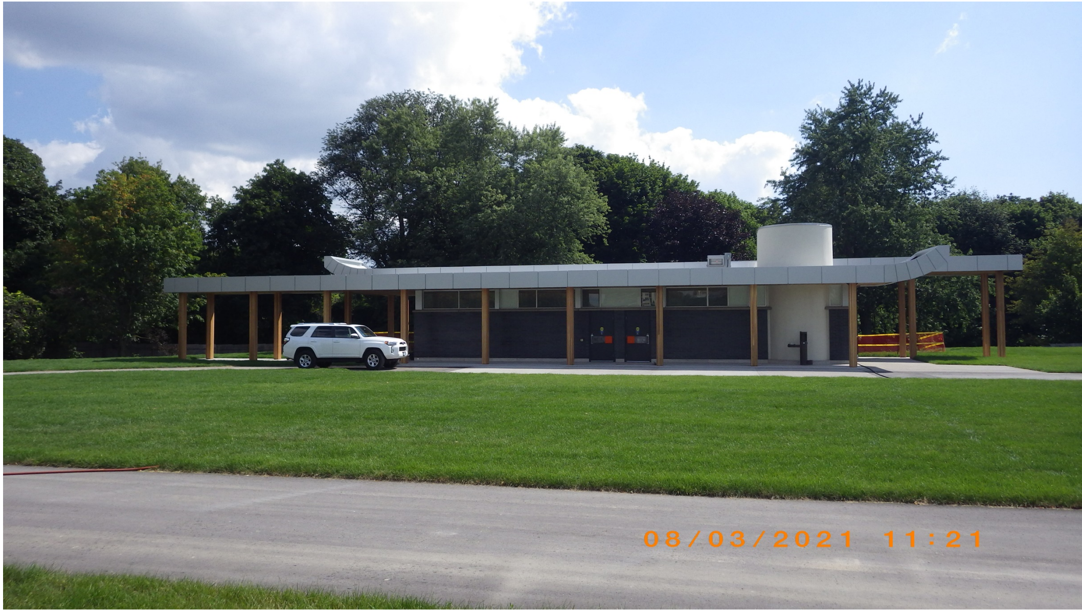
Washroom – west view
