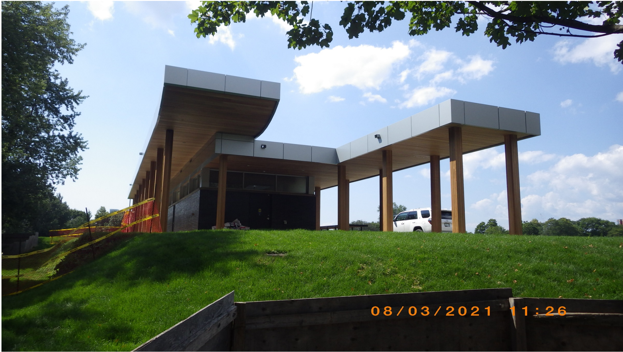
Washroom – north view
