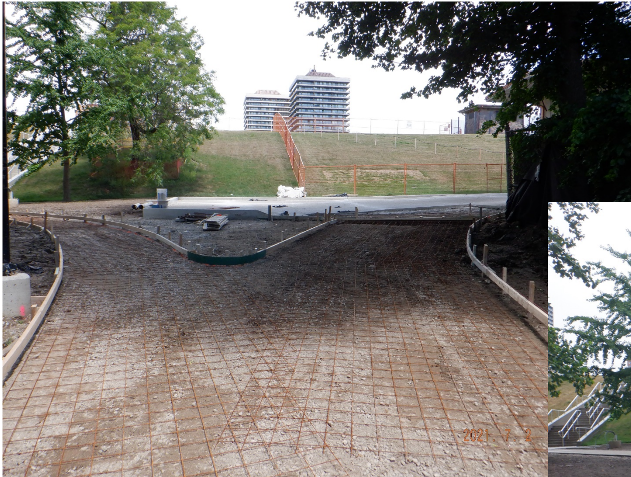
Little park driveway - forms
