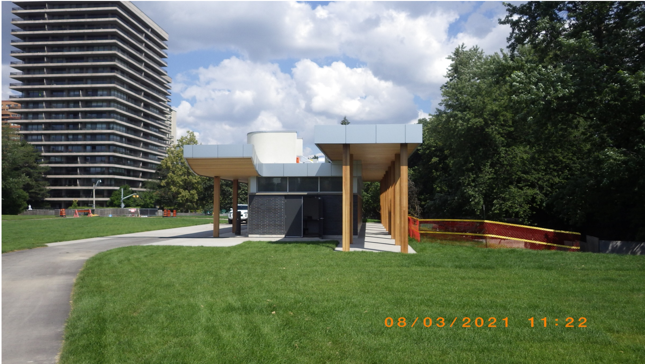
Washroom – south view
