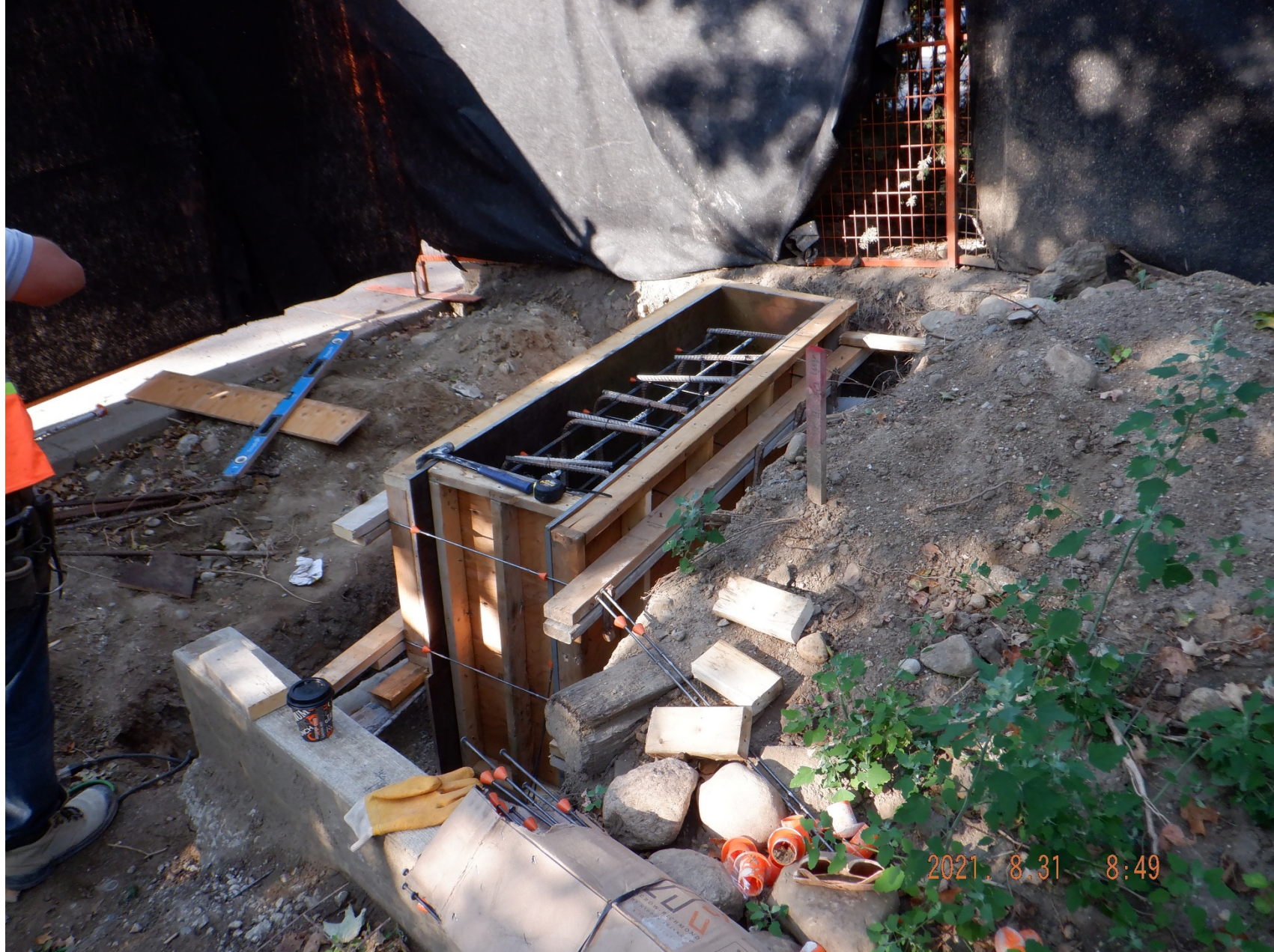
The footings for the community bulletin board located in Little Park/Summerhill Entrance
