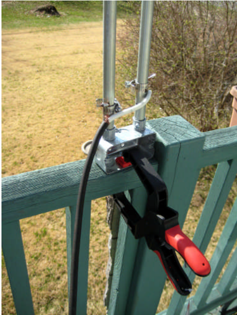
The feed line attached with hose clamps.
