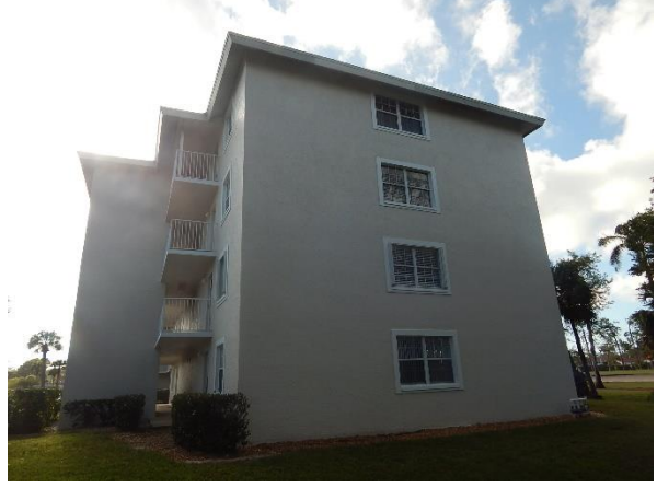
View of north elevation.
