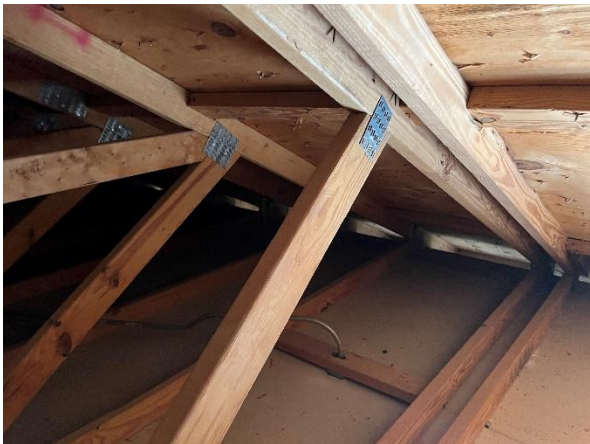
View of roof trusses and decking.
