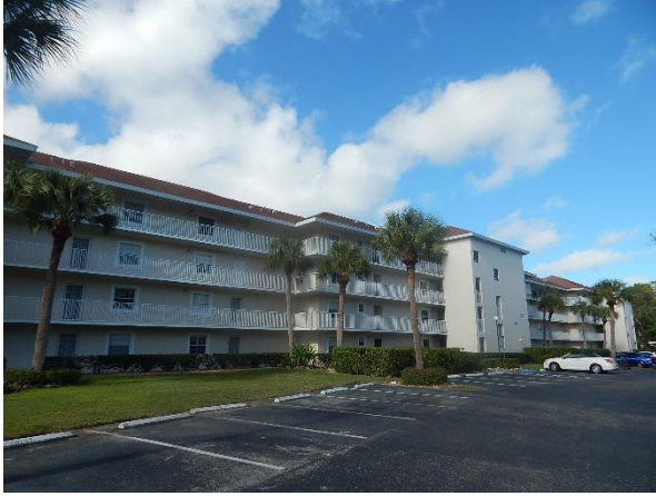
View of front of building.
