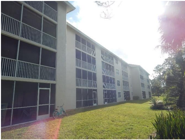
View of rear of building.
