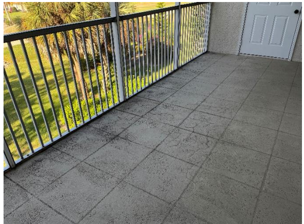
View of typical balcony.
