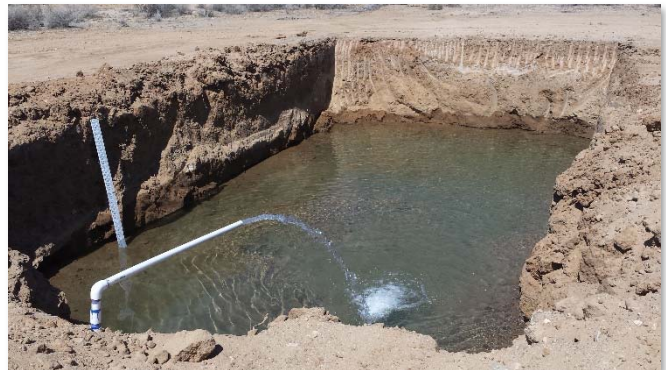
Example: Infiltration Test in Alto Subarea, Mojave Water Agency (manual flow control and water level monitoring)
