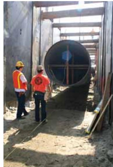
*A segment of the 78-inch-diameter Central Feeder, Phase 1 pipeline is lowered into place.*
