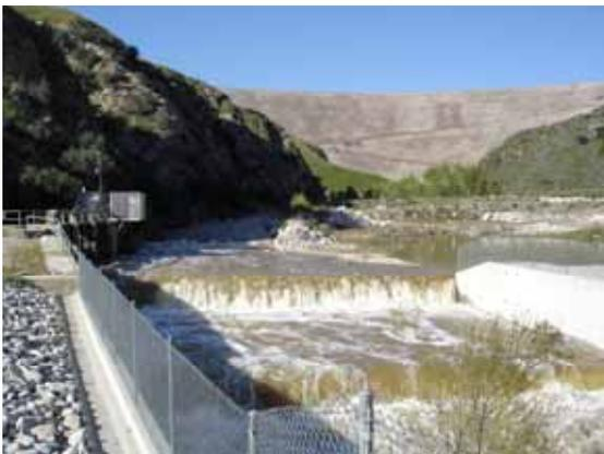
*The Cuttle Weir is a concrete and rock diversion structure owned by the San Bernardino Valley Water Conservation District and is used to divert water from the Santa Ana River to the Conservation District’s Santa Ana River Spreading Grounds for artificial recharge of the SBBA. The Seven Oaks Dam can be seen in the background. The good quality Santa Ana River water is used to recharge SBBA, hence improving water supply reliability and improving SBBA groundwater quality.*
