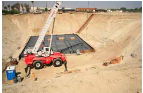
*Foundation for the Redlands Pump Station which will deliver water into the Central Feeder, Phase 1 Pipeline.*
