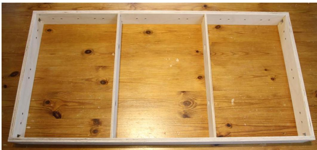
Assemble the frame WITHOUT GLUE to check it fits perfectly.
