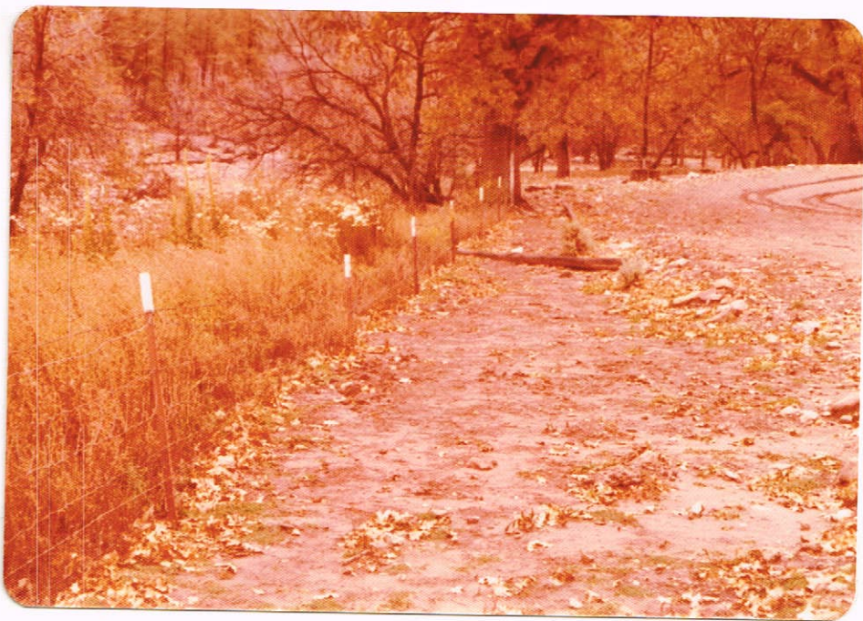
Figure 10. Since this fence was constructed in 1960, sediment from the adjacent hillside (in Naegelin Canyon) has buried much of its lower half.
