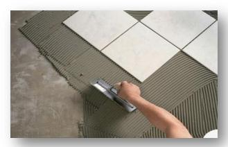
Multipurpose highly polymer modified and very highly deformable adhesive for installation of very large format tiles on most of the substrates to accommodate movements. It offers exceptionally good handling properties with good sag and slump resistance. It can be applied up to 15 mm bed thickness.
