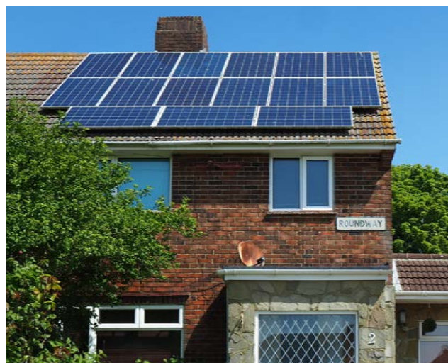
PV panels integrated into the roof of a dwelling within Coldean.
