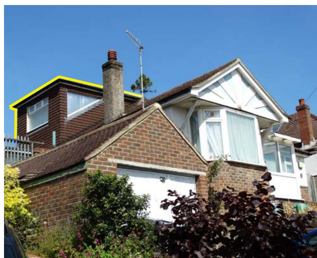
Example of a dormer extension (yellow) that is commonly observed within Coldean which is of an appropriate orientation, alignment and scale that complements the original roof.
