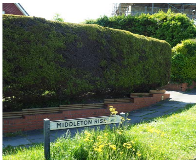
Low-rise brick and timber boundary wall with a well-defined hedgerow placed adjacent to a green verge. These materials are complementary to the vernacular within Coldean.
