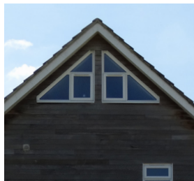
Triangular windows aligned to roof pitch
