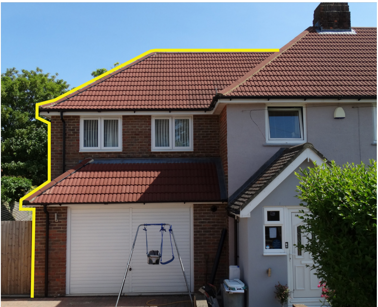
Example of a double-storey side extension (yellow) that complements the height, roof type and materiality and window alignment of the original building.
