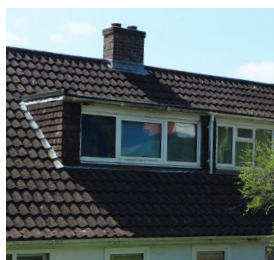
Double-width flat roof dormer
