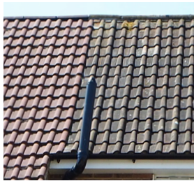
Overlapping clay Gaelic roof tiles
