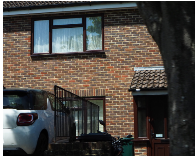
Fenestration using a timber frame or colour that is fitting with Coldean's palette can enhance the street scene.
