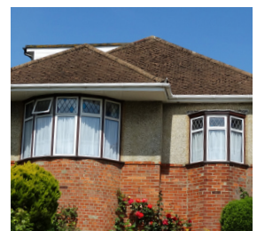
Bow window (left) aligned with bay window (right)
