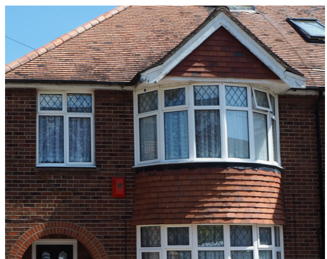
Consistent patterned muntins on the top half of the windows consistent throughout the entire street facing facade.
