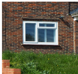
Casement window opening on side and top
