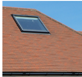
Simple red clay roof tiles
