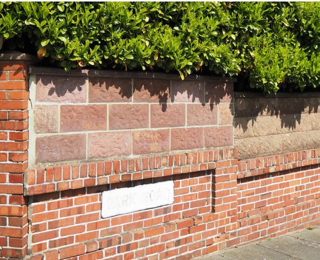
Mix of boundary treatment materials with a consistent colour palette. This mix of hard and soft boundary treatment is easier to maintain than a wholly soft boundary treatment and adds variance.
