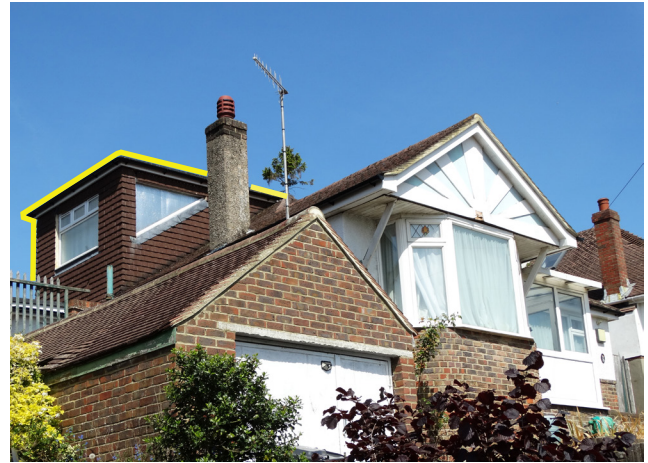
Example of a side dormer extension (yellow), which is of an appropriate orientation, alignment and scale that complements the original roof.
