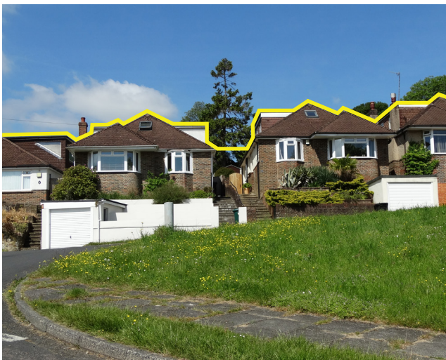
Consistent roofline between neighbouring dwellings including a uniform dormer extension style.
