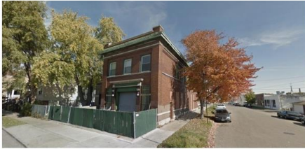
The Plant Vertical Farm - Chicago
