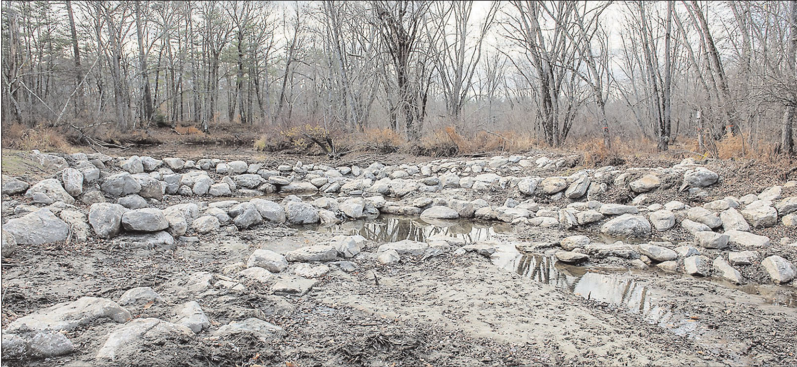
Gradient rock ledges, seen Nov. 7, were installed to allow a continuous flow of water throughout the year, but beaver dams have stopped nearly all the water flowing from Hogan and Whitney ponds into the Little Androscoggin River in Oxford. RUSS DILLINGHAM/SUN JOURNAL
