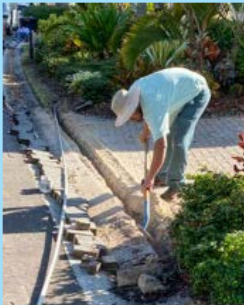
Conduit & wire being installed
