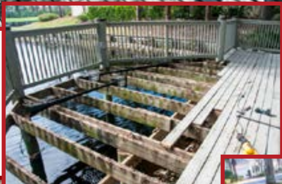
New joists added
