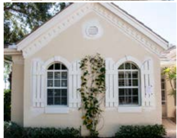
Trim painting prior to stucco painting
