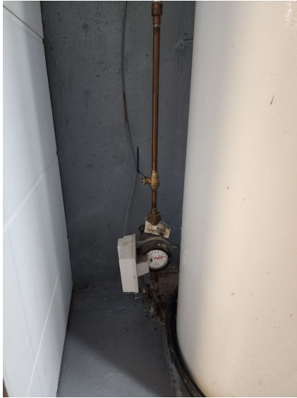
Main water shut off
