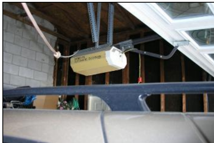
17. Extension cord for west garage door opener
