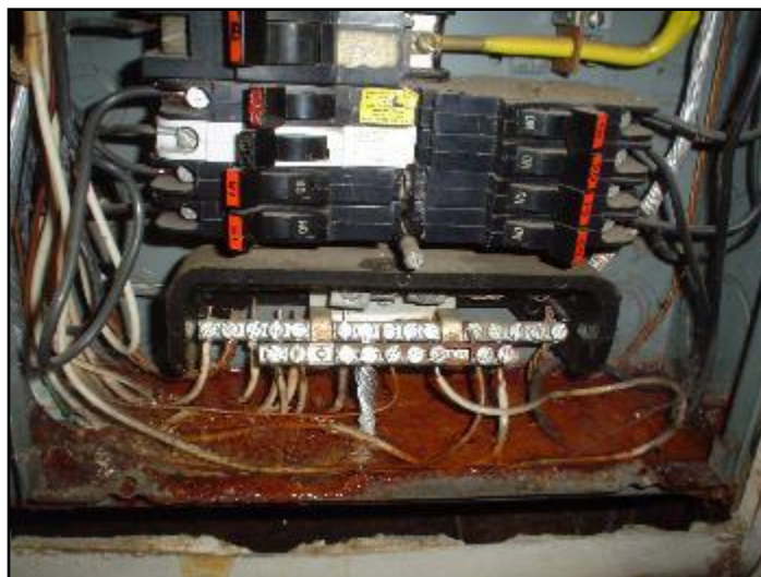
7. Water and rust in bottom of panel
