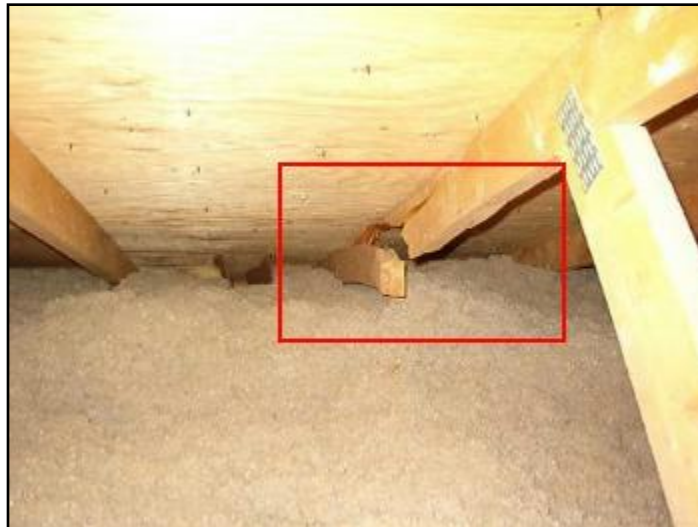
6. Top chord of truss is broken
