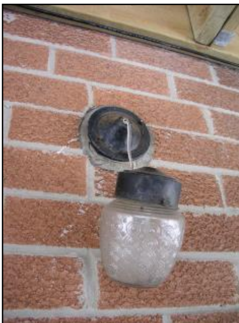
8. Light fixture is not well secured
