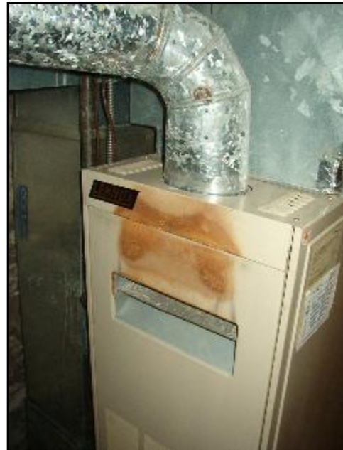
10. Evidence of furnace backdrafting
