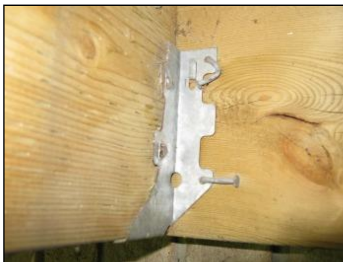
4. Poor end bearing, joist hanger connections
