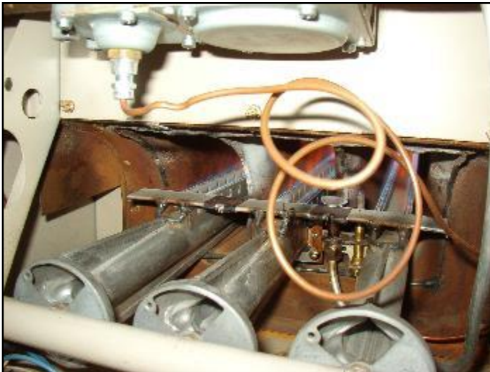
9. Rust at bottom of heat exchanger
