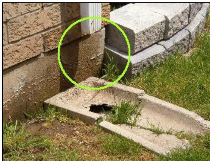
3. Downspout ends too close to building
