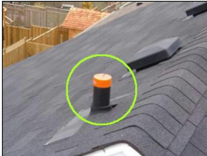
15. Plumbing stack is capped
