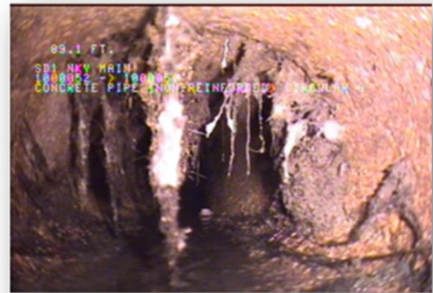
Figure 2. The CV model predicted Pipe Collapse (XP) and Root Fine Joint (RFJ) defects that were missed by humans
