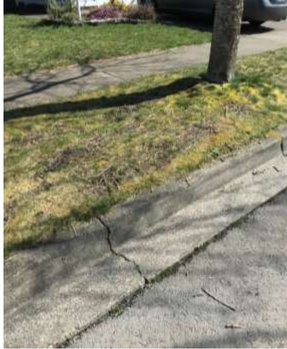
Photo of Typical Damage with Red Maple
