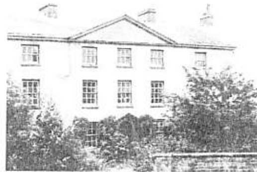
The dilapidated Rectory
