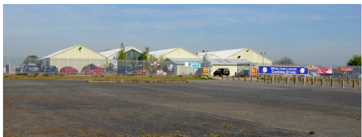
Whilton Locks Garden Centre and tarmac area from Nobottle Road
