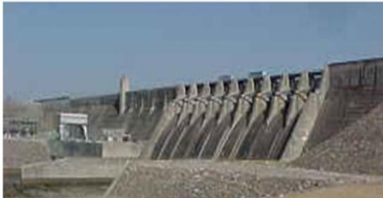
principal of this type of structure is to provide as watertight a structure as possible to prevent loss or leakage of water through or around the structure. This is accomplished by making the foundation of the dam consist of concrete and the dam itself is a concrete structure. The dam consists of concrete blocks and is located in the original river channel. The
