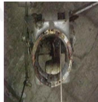
**Note:** Proper release of the hanger should be to raise the gate a small distance to relieve the pressure on the hanger, then pull the chain down to open the hanger, releasing the coned head.
