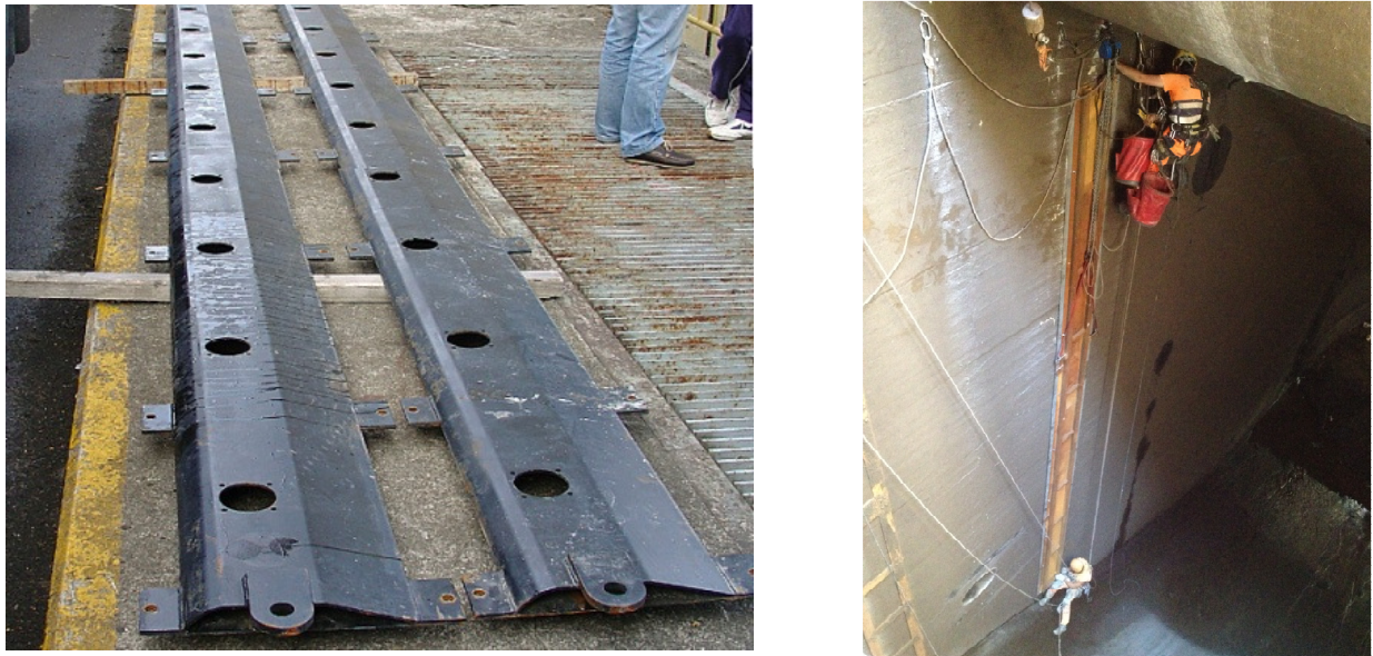
Fig. 4 – ASFM frame in the yard (left) and in the intake bay (right)
