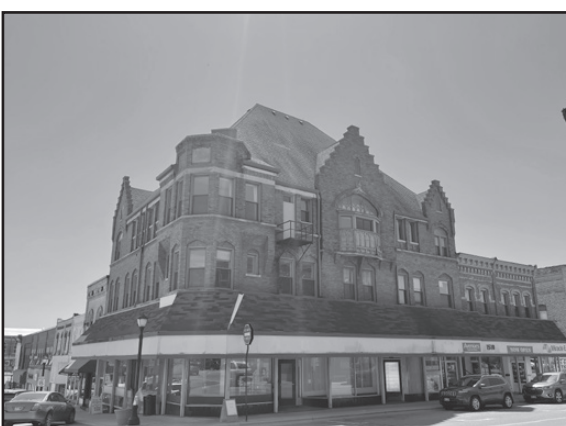
White Building prior to project
