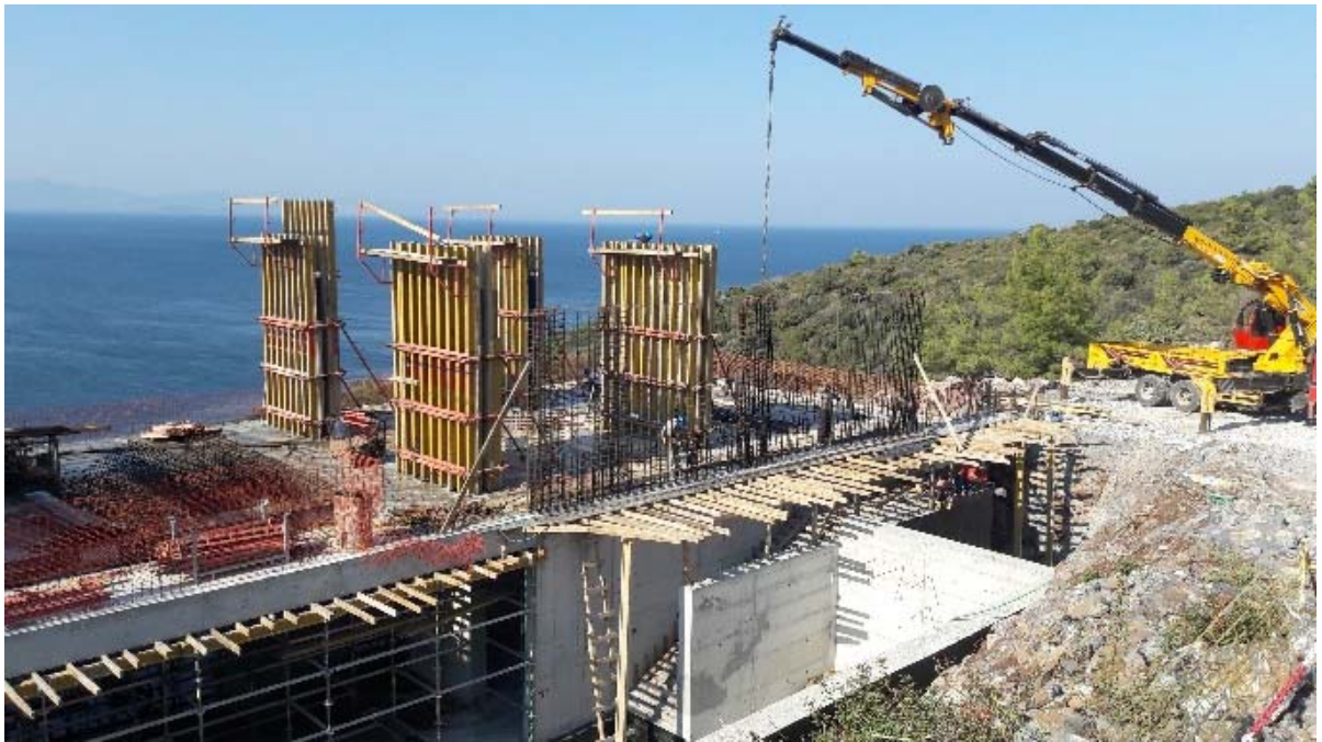
Construction of a new villa complex at Kaplankaya, Mugla, Turkey.
