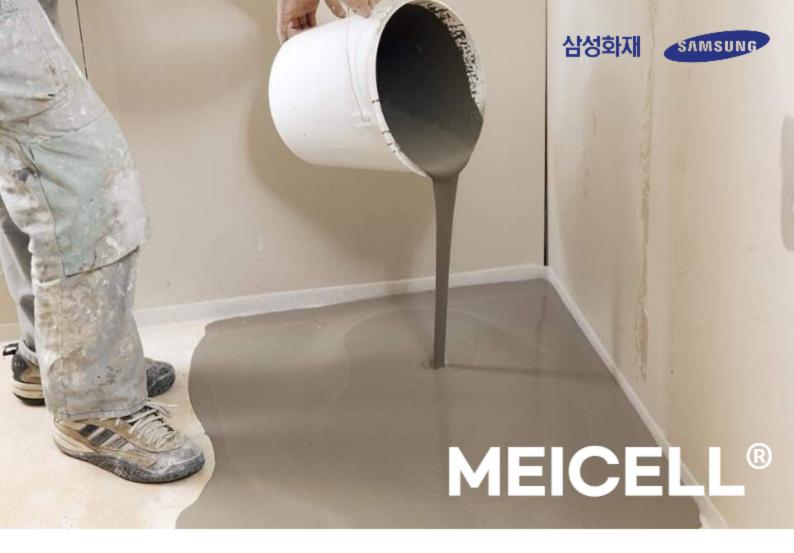
Self-leveling mortar can form a flat, smooth and strong foundation on the substrate by its own weight, so that other materials can be laid or bonded, and large-area and high-efficiency construction can be carried out.
