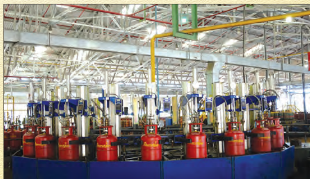
LPG Bottling Plant
