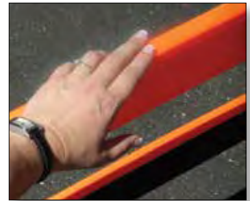
The top panel acts as a smooth continuous guide for the hand
