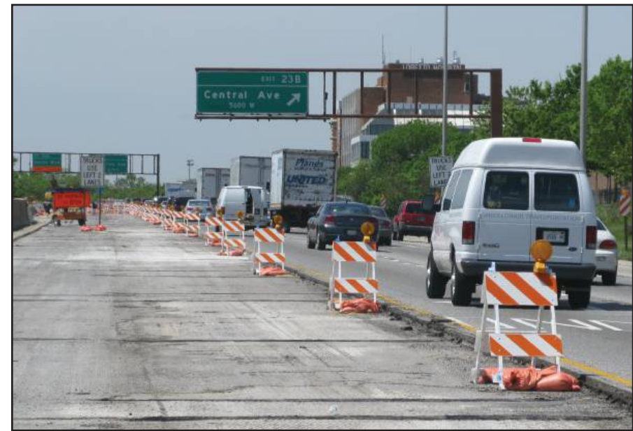
Fibercade™ Barricades on the Eisenhower Expressway - Chicago, IL
