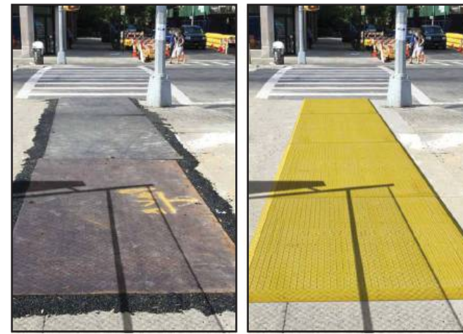
Steel Plates with Cold Patch
