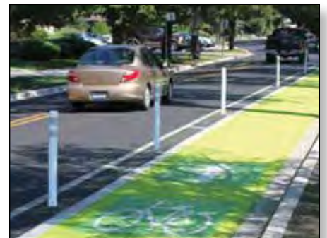
Bike lane and pedestrian walkways
