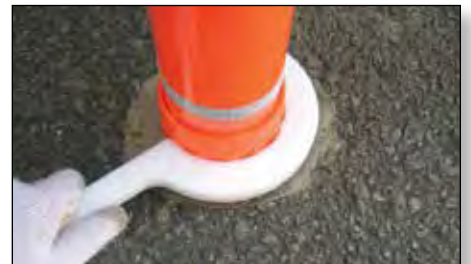
City Posts can be tightened and loosened with the City Post wrench
