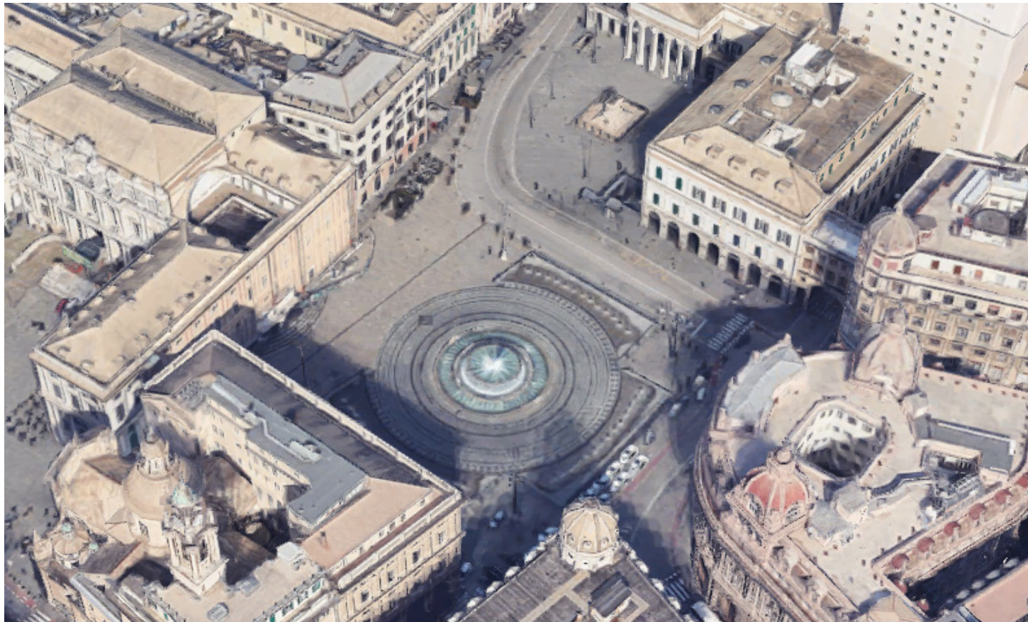
WATER COOLING Exterior Temperature Moderator
