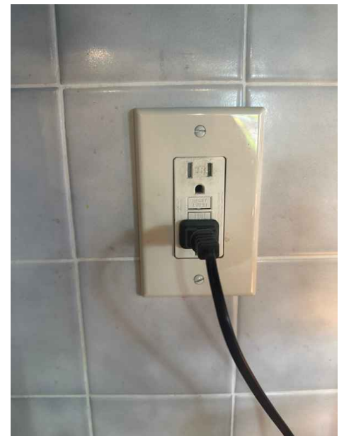
GFCI & AFCI: GFCI Protection Yes - Functional, GFCI Receptacles GFCI receptacles in kitchen only. Bathrooms are on GFCI breaker.
