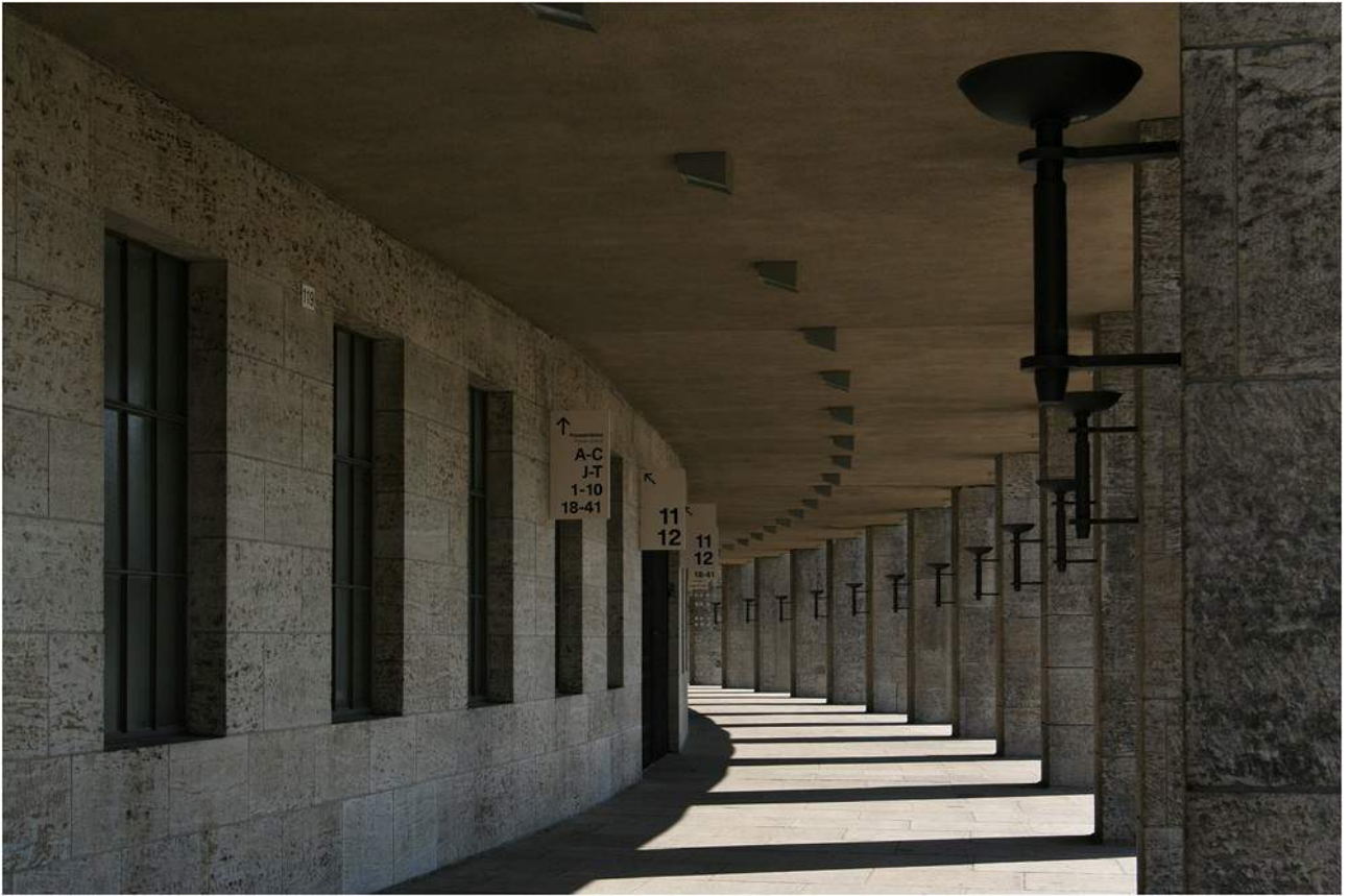
Above: Olympiastadion Berlin (1936, 2006). Preservation of exterior historical character-defining elements.
