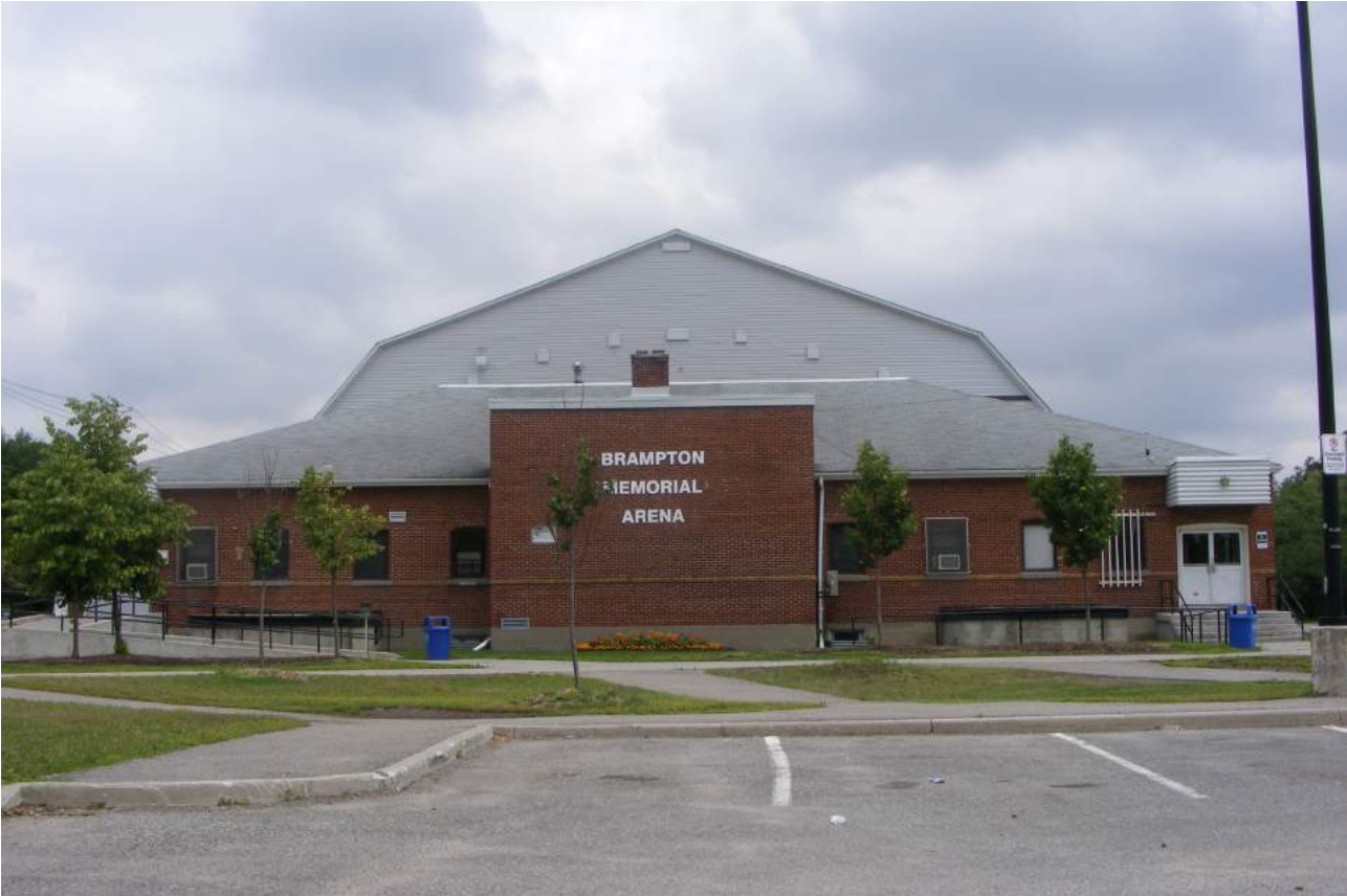
Brampton Memorial Arena – Brampton, Ontario (1950)
