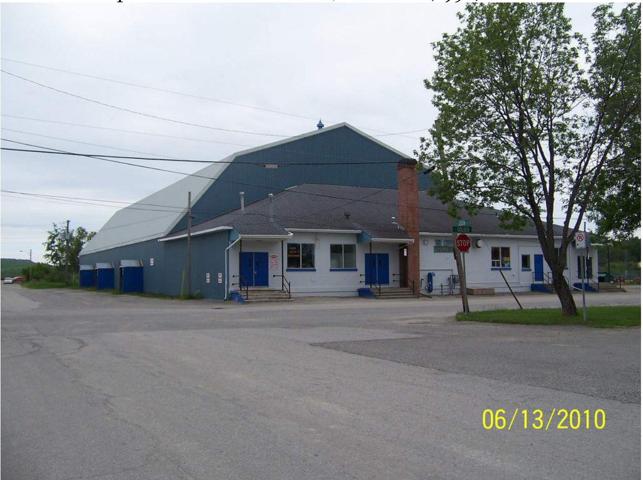
South Porcupine Arena – Timmins, Ontario (1930)
