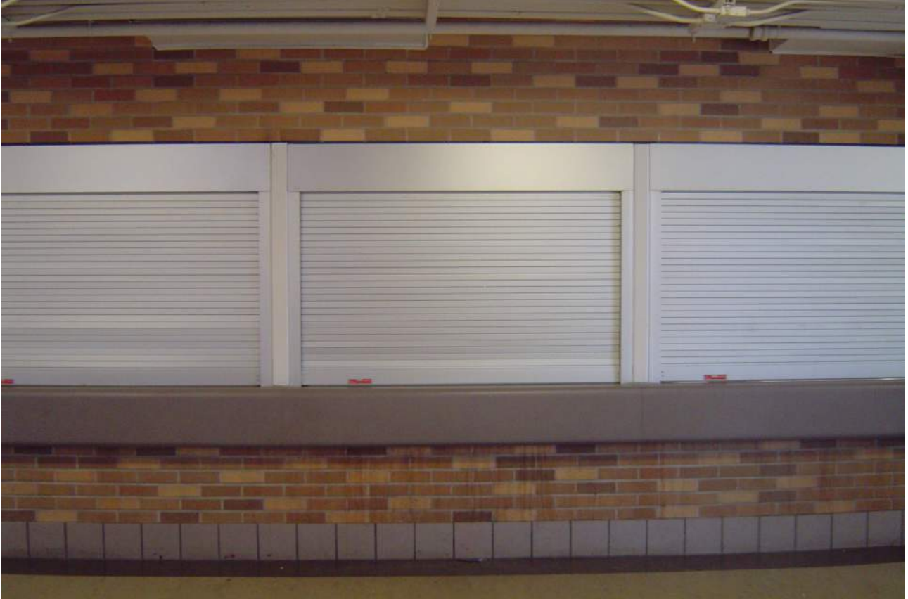
Below: Galt Arena Gardens, replacement ticket booth
