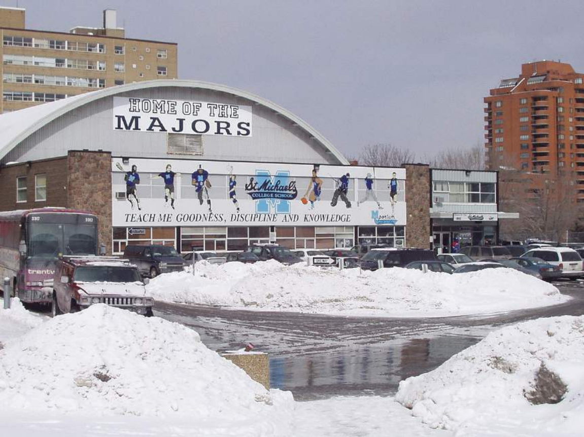
St. Michael's College School Arena – Toronto, Ontario (1961)
