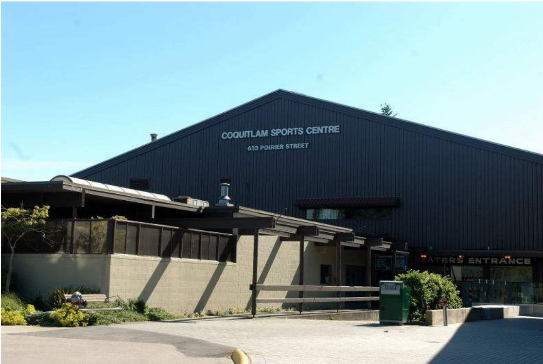
Coquitlam Sports Centre – Coquitlam, British Columbia (1961)
