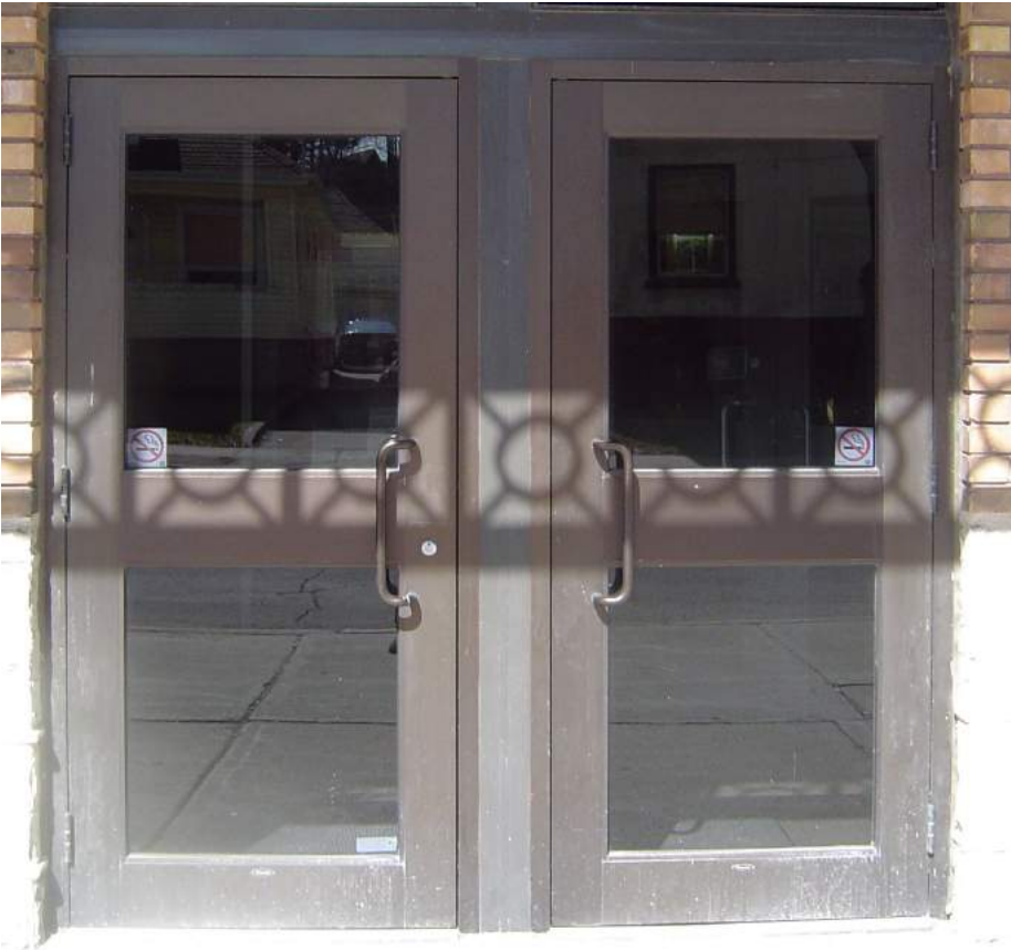
Below: Galt Arena Gardens, replacement doors
