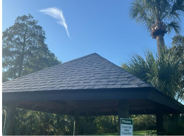
Pavilion shingle roof
