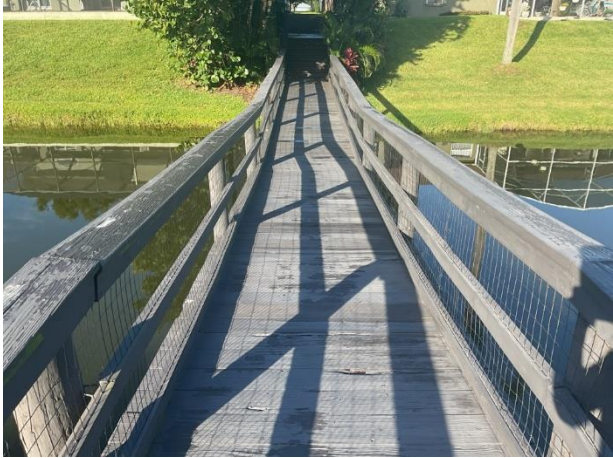
Wooden bridge overview
