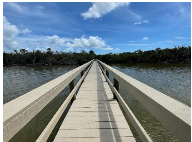
Dock with wood decking
