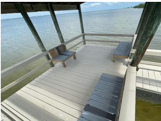
Dock with wood decking
