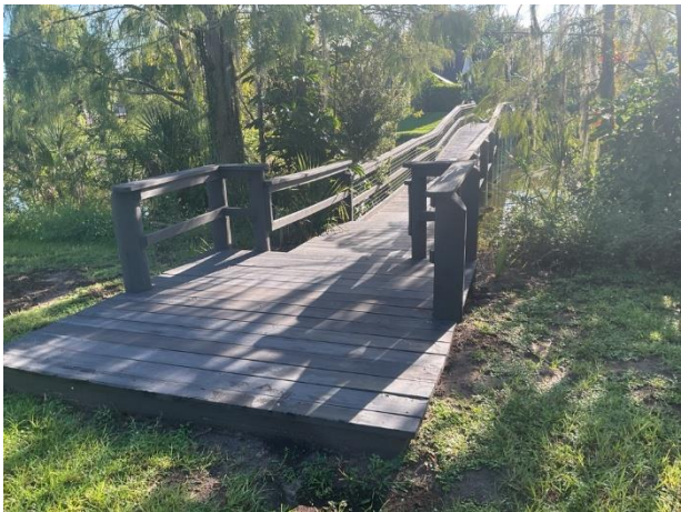
Wooden bridge overview
