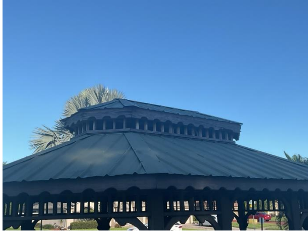
Gazebo metal roof
