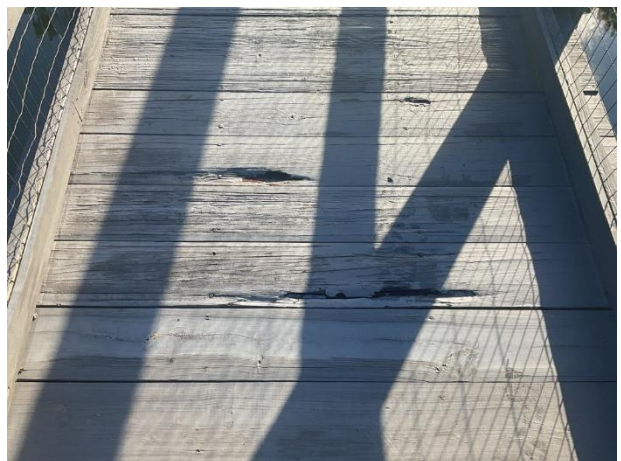
Wood deterioration
