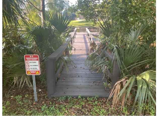
Dock with wood decking
