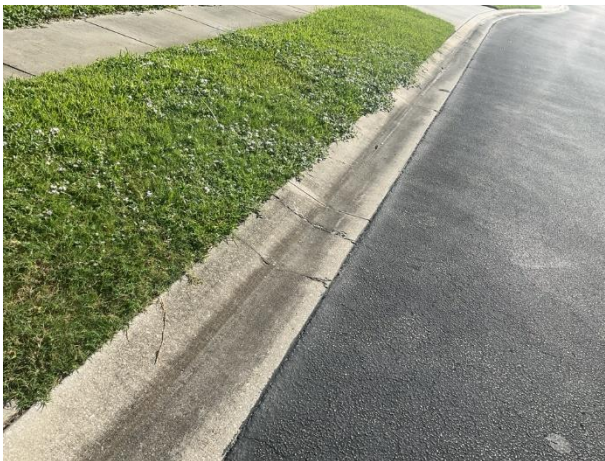
Concrete curb and gutter
