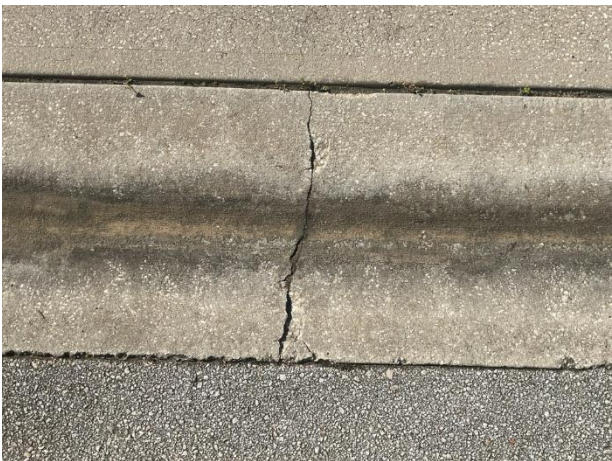
Concrete cracks
