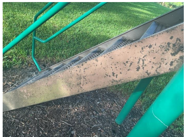
Playground equipment with biological growth
