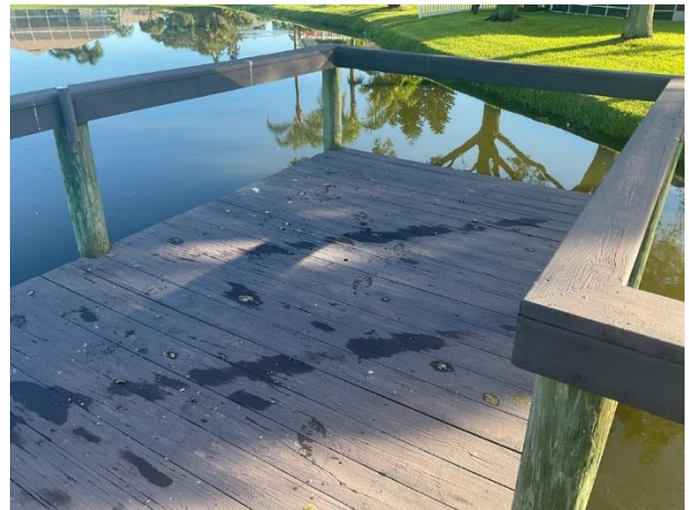
Dock with wood decking
