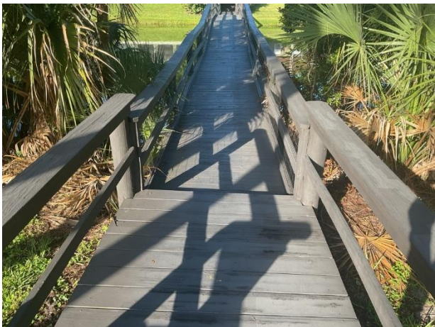
Wooden bridge overview
