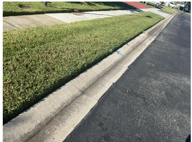
Concrete curb and gutter
