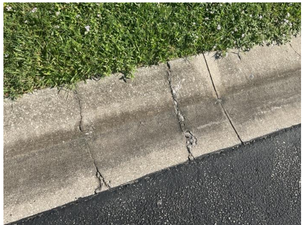
Concrete cracks
