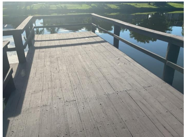
Dock with wood decking
