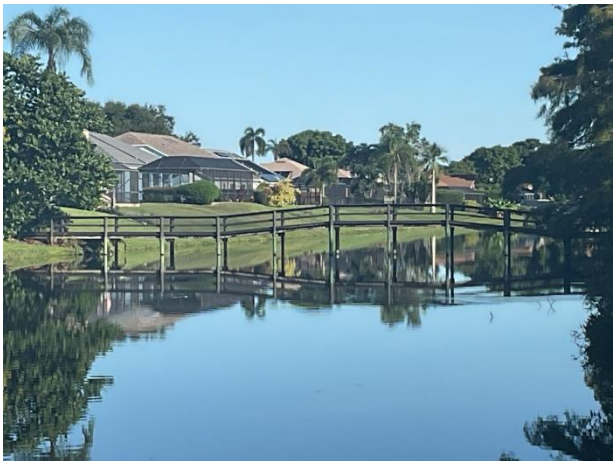
Wooden bridge overview
