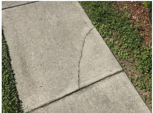
Sidewalk cracks
