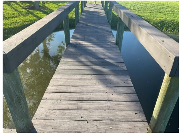
Dock with wood decking
