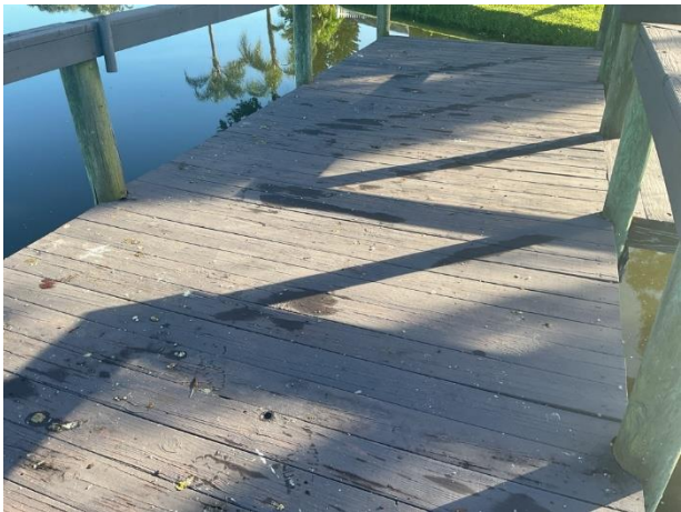
Dock with wood decking
