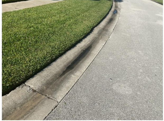
Concrete curb and gutter
