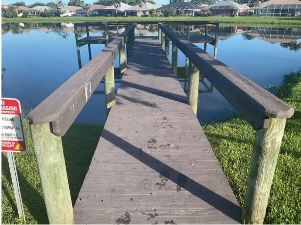
Dock with wood decking
