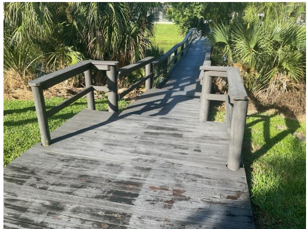
Wooden bridge overview
