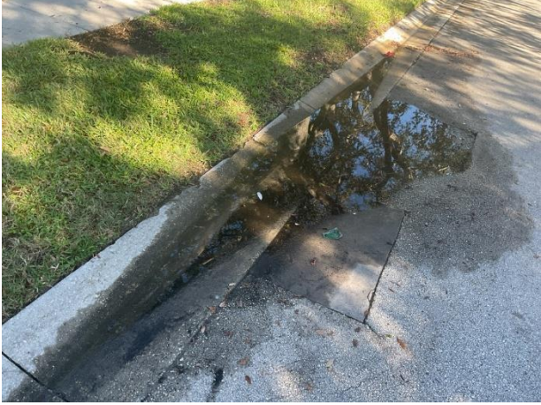
Concrete curb and gutter kilarney
