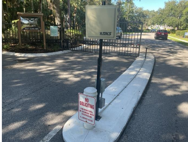
Gate entry barcode scanner
