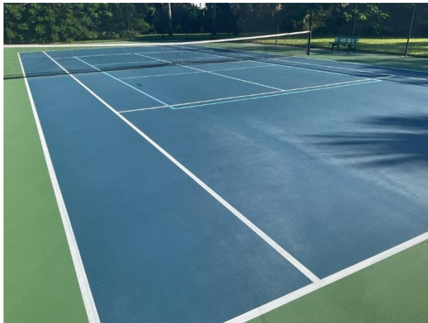
Tennis court overview
