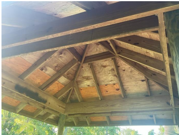
Pavilion roof structure
