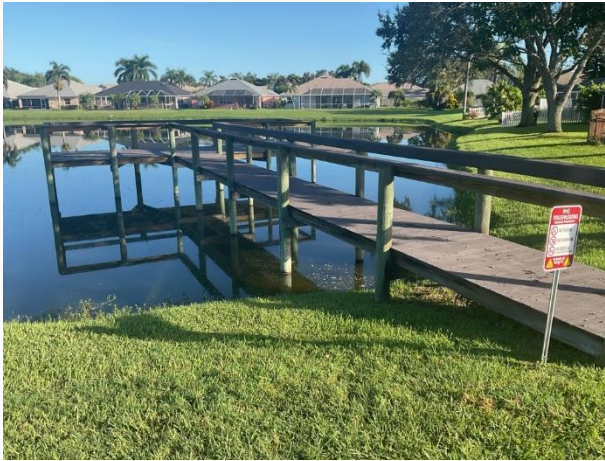
Dock with wood decking
