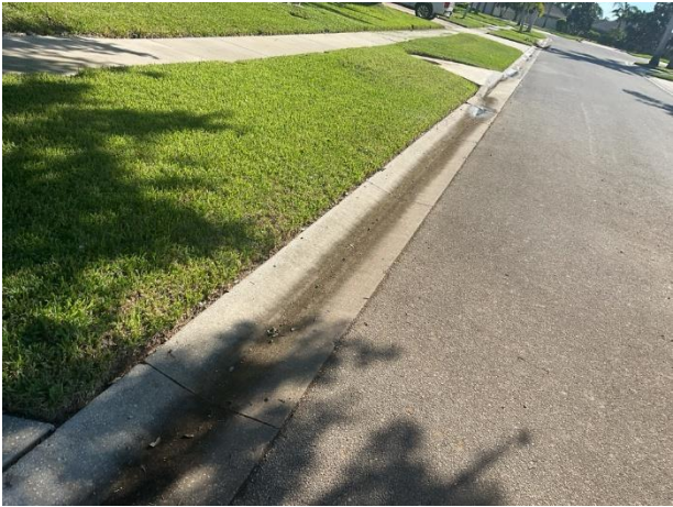
Concrete curb and gutter
