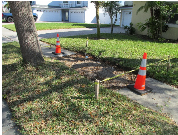
Concrete sidewalks with replacements underway
