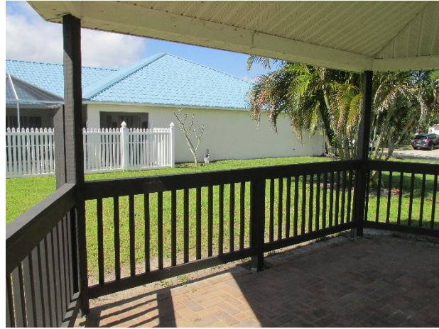
Gazebo paver deck, railings and soffit
