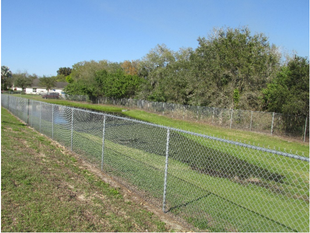
Chain link fence
