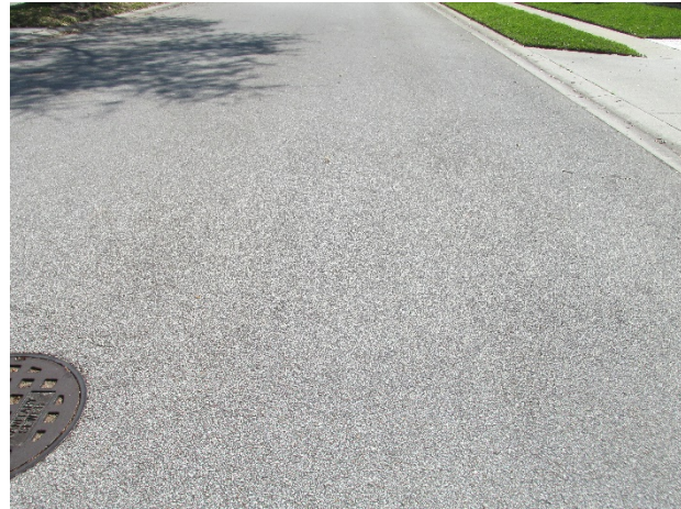
Asphalt pavement on Limerick Drive
