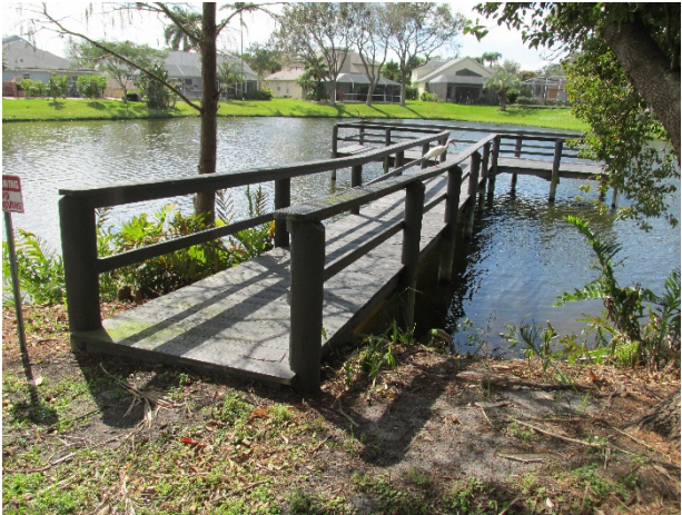
Wood dock overview
