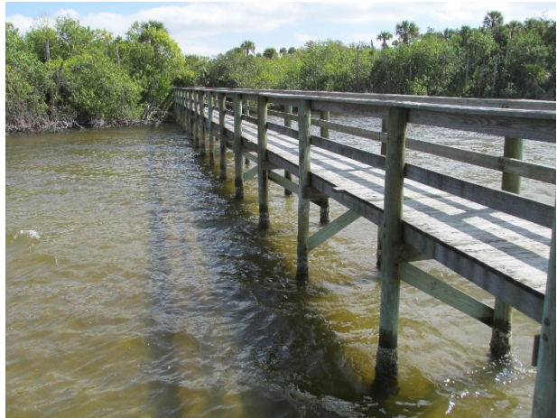
Wood pier overview
