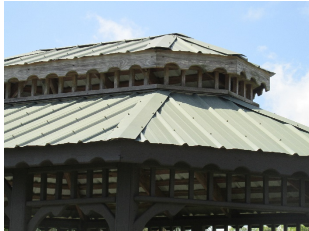
Gazebo metal roof
