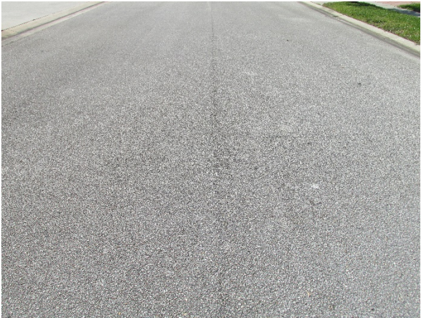
Asphalt pavement on Tipperary Drive
