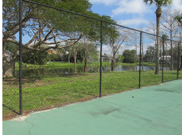
Tennis court fence
